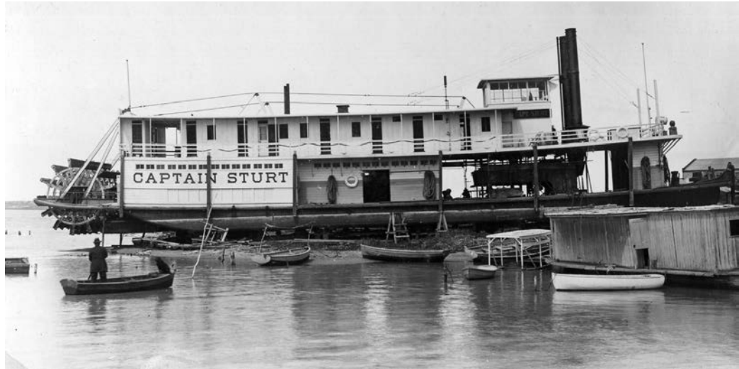
PS Captain Sturt under construction, 1915. Photo: SA Water, Book 088 page 137 image 425.
