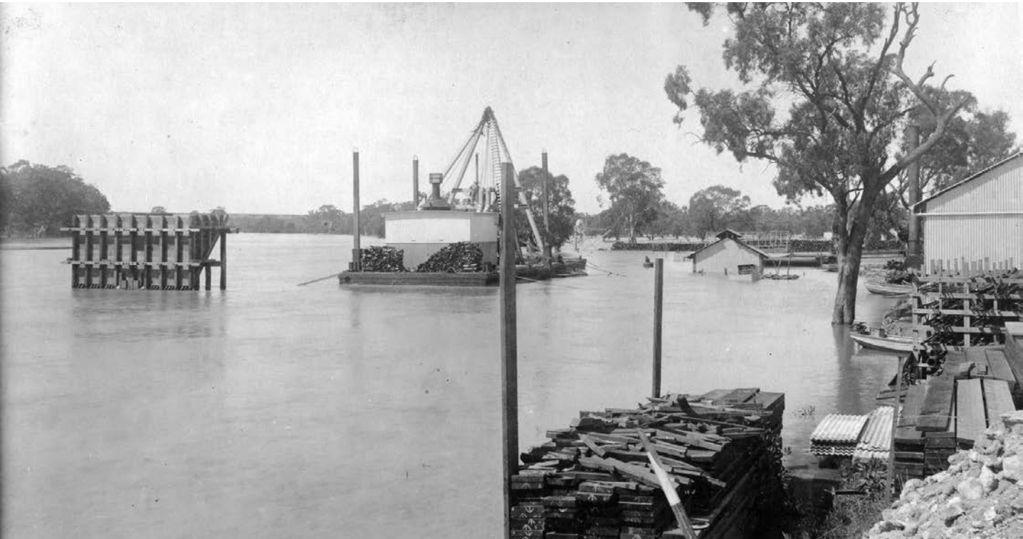
Blanchetown flood 1917, showing worksite buildings and plant inundated. Cofferdam completely submerged.
